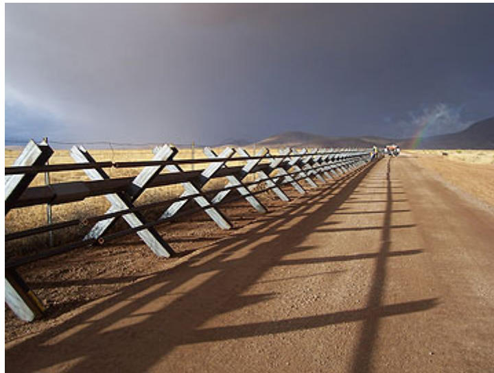
Figure 8. Vehicle fencing outside of El Paso 240
