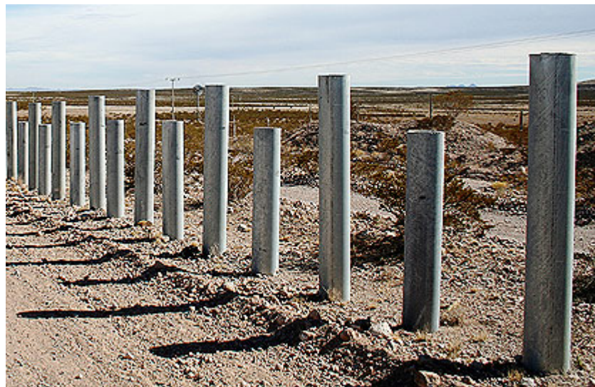
Figure 9. Vehicle Bollards outside El Paso 241
