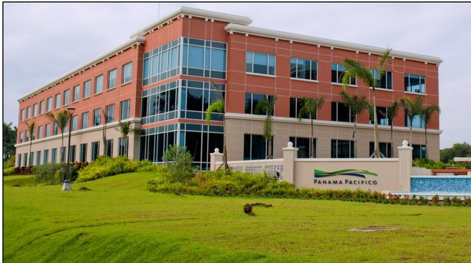
Figure 12. Office building at Panama Pacifico 216
