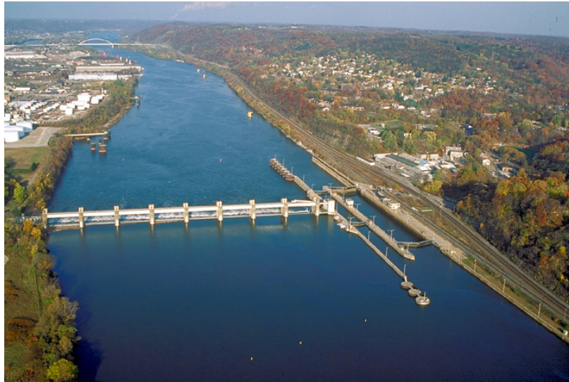
Figure 6. Aerial view of Emsworth Lock and Dam, Pittsburgh, PA. There are two parallel locks (at right) that allow passage between the pools of water separated by the dam (at left). Source: USACE 2012.
