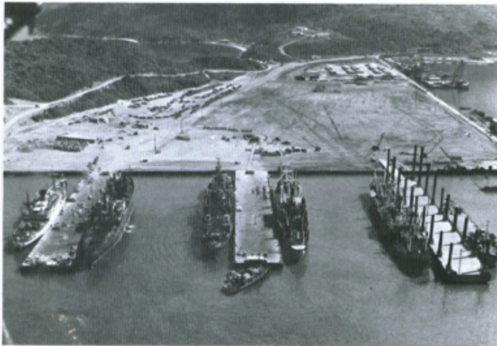
Figure 11. Aerial view of the deep water piers in the Danang Harbor. The DeLong pier can be seen on the right. (Figure 21 in [6])
