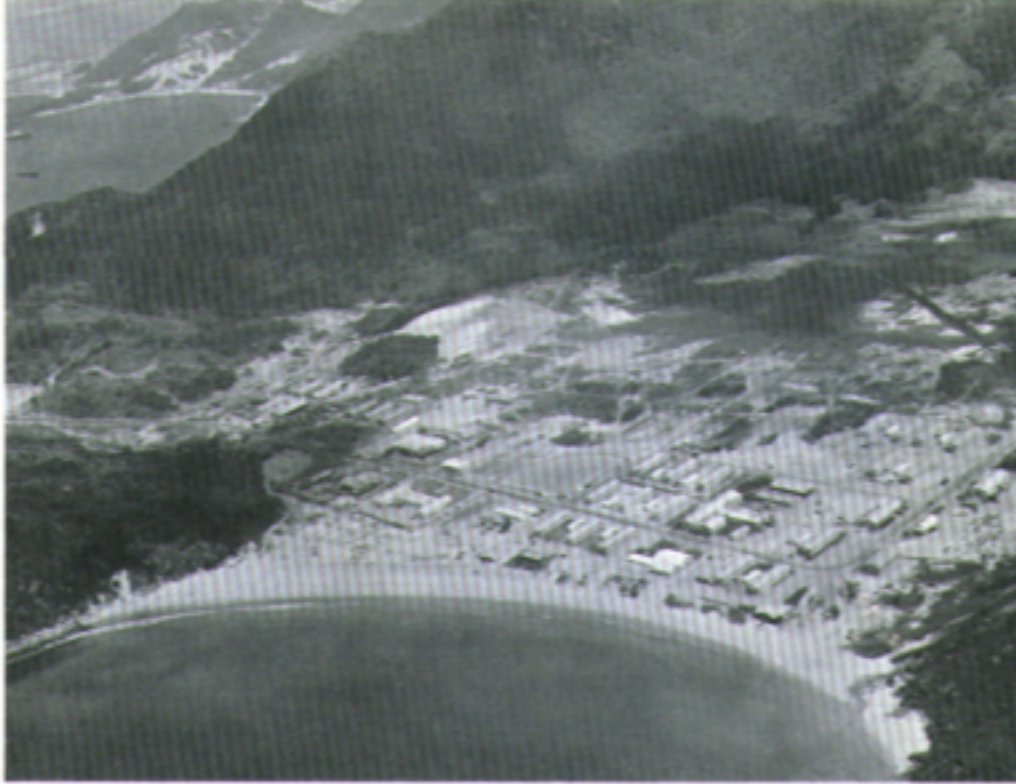
Figure 5. Aerial view of Naval Support Facility, Cam Ranh Bay, 1969. (Figure 12 in [5] courtesy of the Naval Historical Center, Department of the Navy.)
