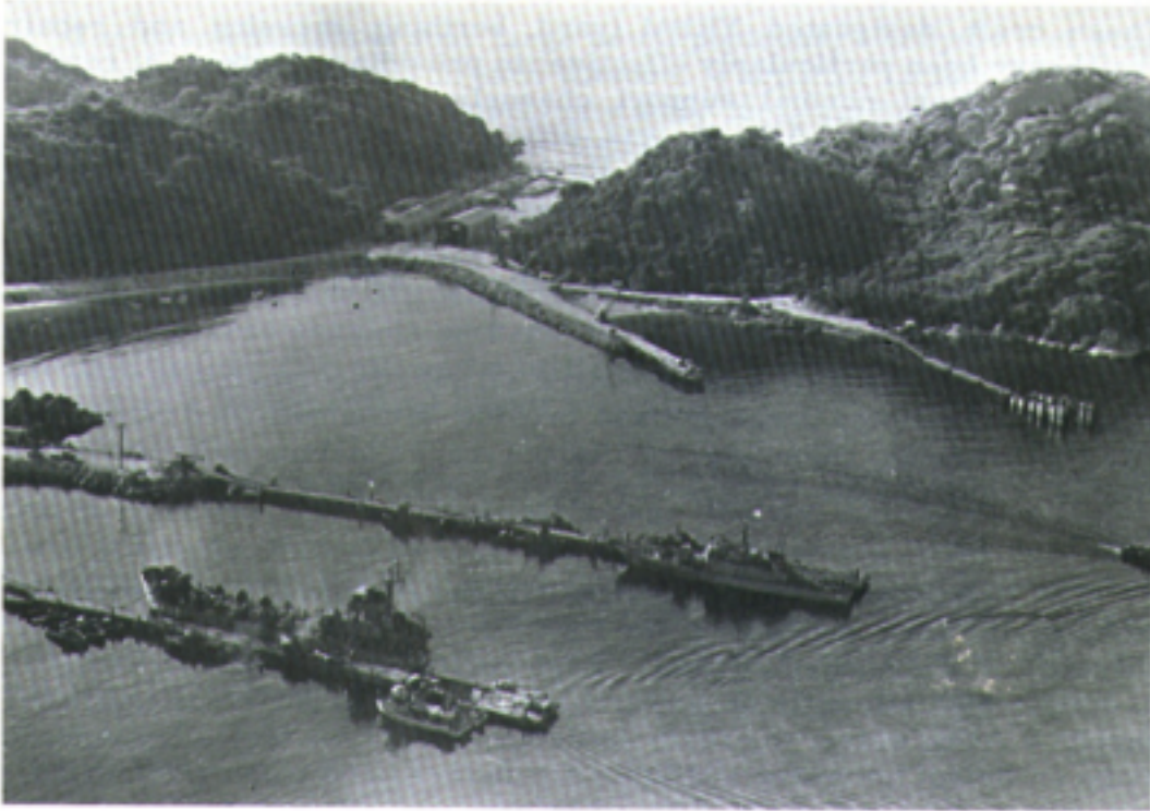
Figure 6. Pontoon piers at the Naval Support Facility, Cam Ranh Bay, 1969. To the far right is a small floating drydock. (Figure 14 in [5] courtesy of the Naval Historical Center, Department of the Navy.)
