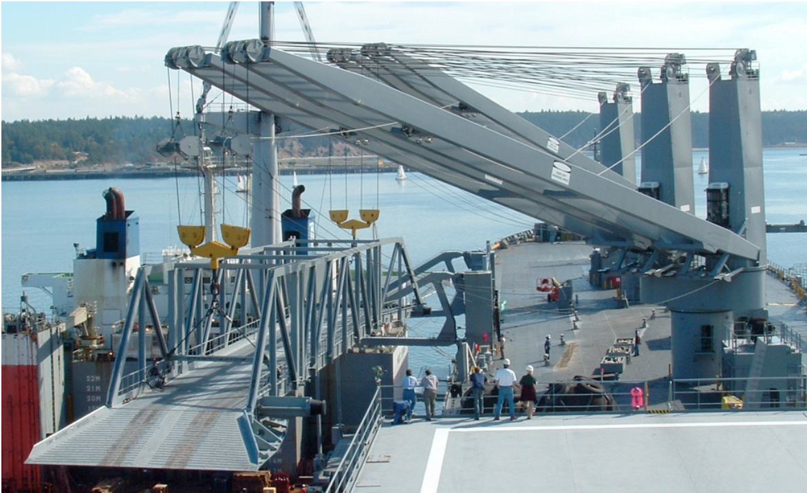
Figure 25. Photo of a sideport ramp of a Large Medium Speed Roll-on/Roll-off (LMSR) vessel being lifted into place by two luffing-jib crane-sets in twin mode.
