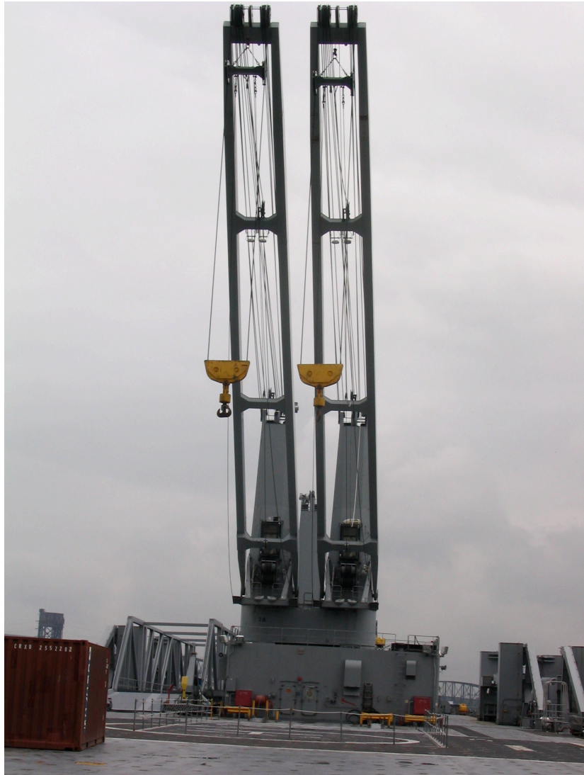
Figure 23. Photo of two luffing jib cranes mounted on a twin platform.
