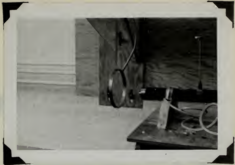
PHOTOGRAPH 9 6" Diameter Ring Anode, Flameholder, and Combustion Tube
