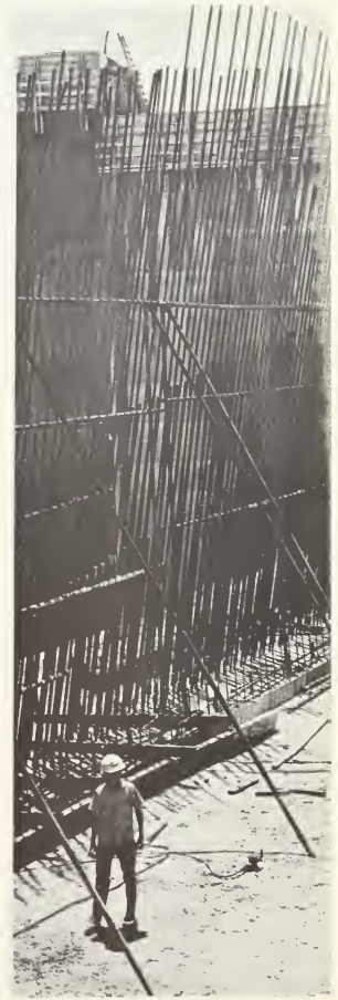
● A worker walks past a row of tall steel rods, which are used as reinforcement in the concrete portion of the dam.
