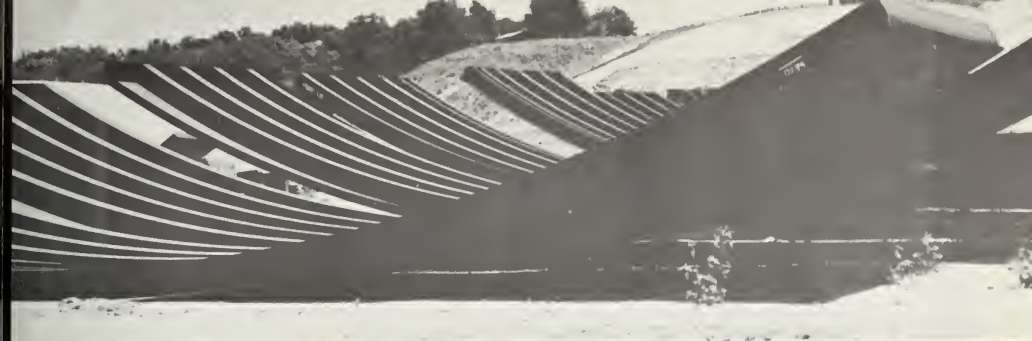
● A worker walks past a row of tall steel rods, which are used as reinforcement in the concrete portion of the dam.
