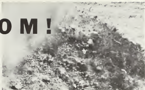
● Exploding dynamite rips the hard rock loose.
