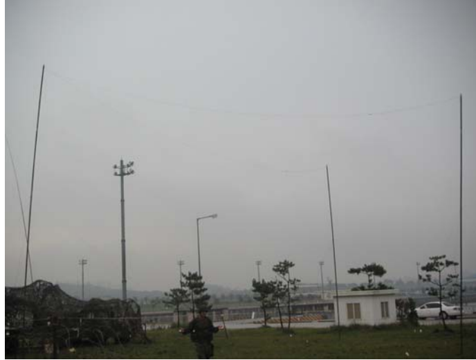
Figure 29. Uchi Focus Lens Sloping Vee Antenna 57
