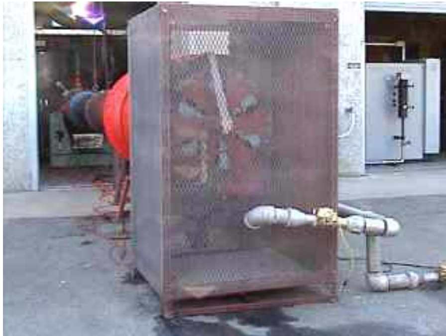
Figure 3. Inlet plenum with steam dump piping, fast acting solenoid, and steam boiler
