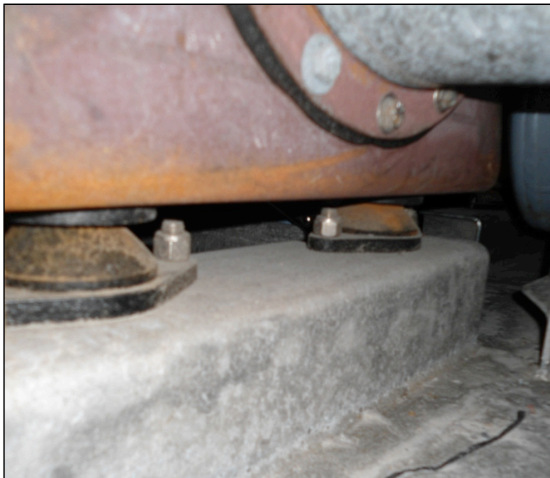
Figure 70: Side View of Vibration Mounts on SENECA.
