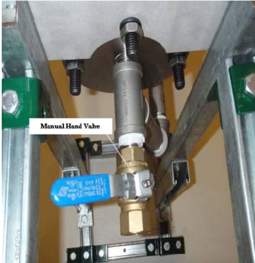
Figure 15. Exhaust System's Flush Valve
