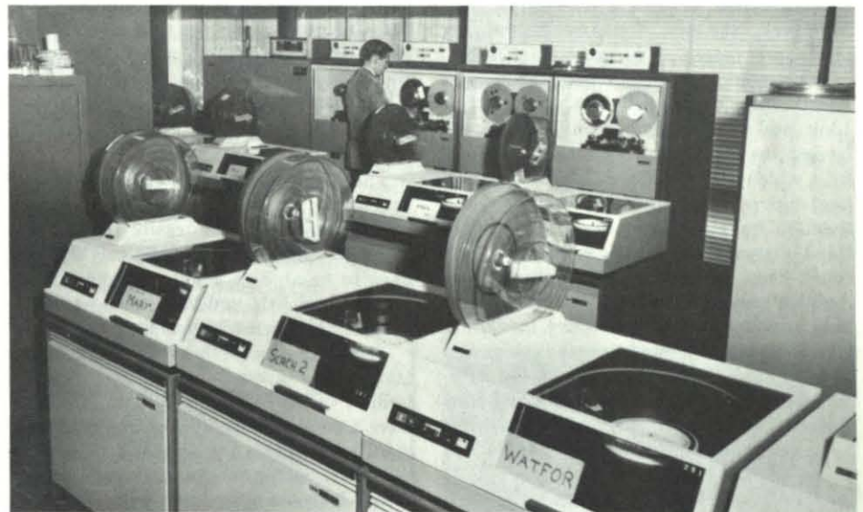
MAGNETIC TAPE UNITS and disk storage units are located in Spanagel Hall.
