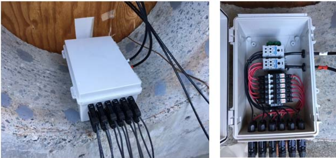
Figure 5. Combiner Box Wiring Configurations.
