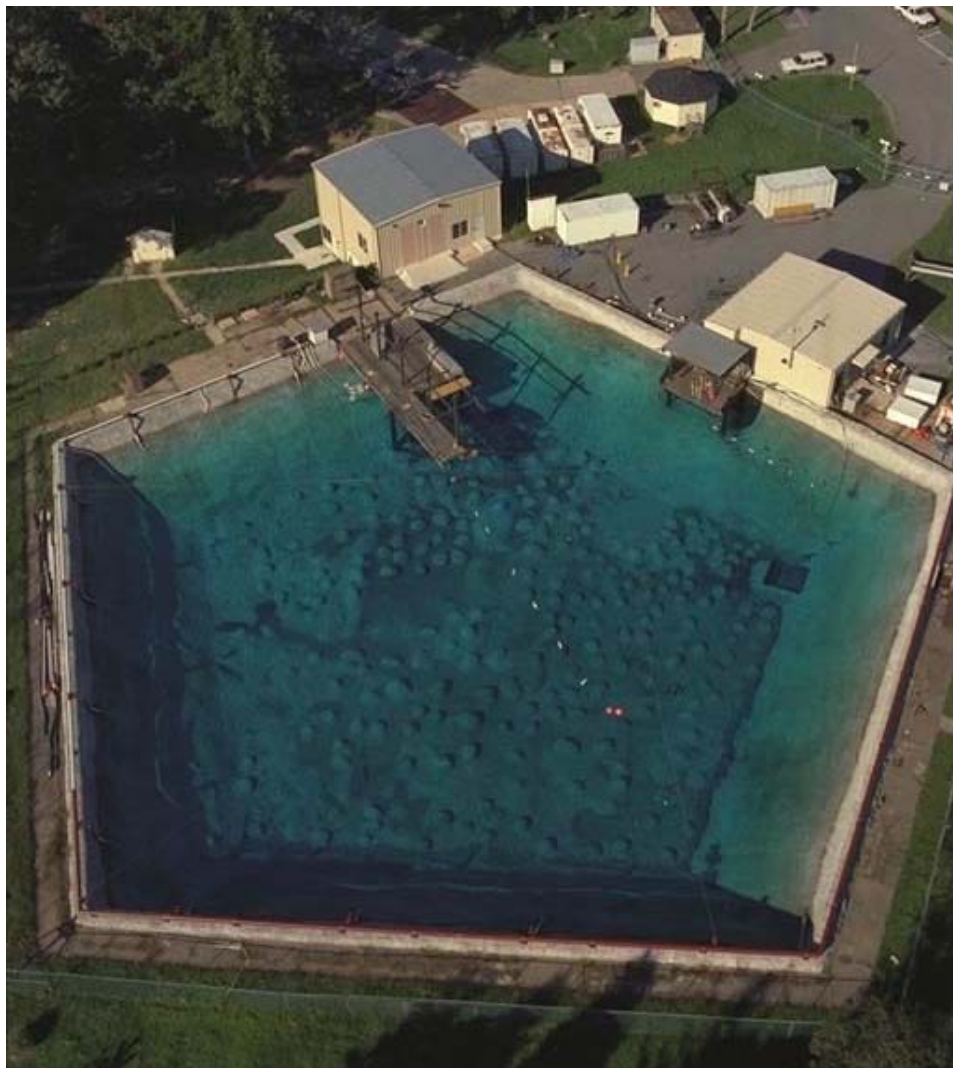
Figure 12. Explosion Test Pond, NSWCCD, West Bethesda, MD. "Photo courtesy of NSWCCD, William Lewis."
