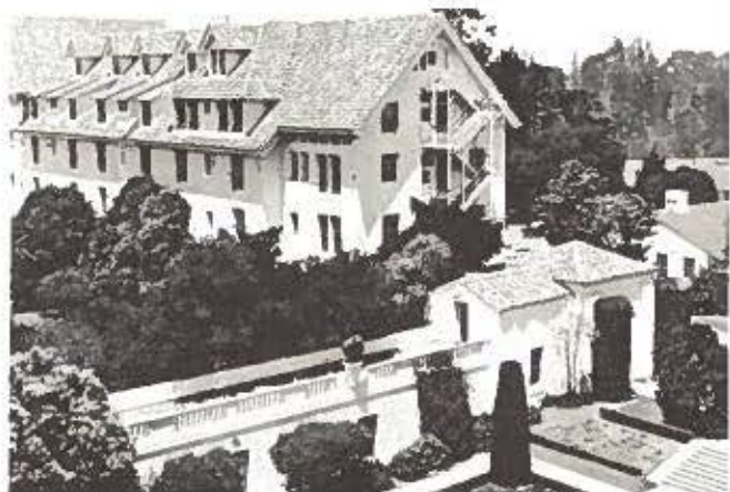
Bldg. 222, housing the General Line and Naval Science School.
