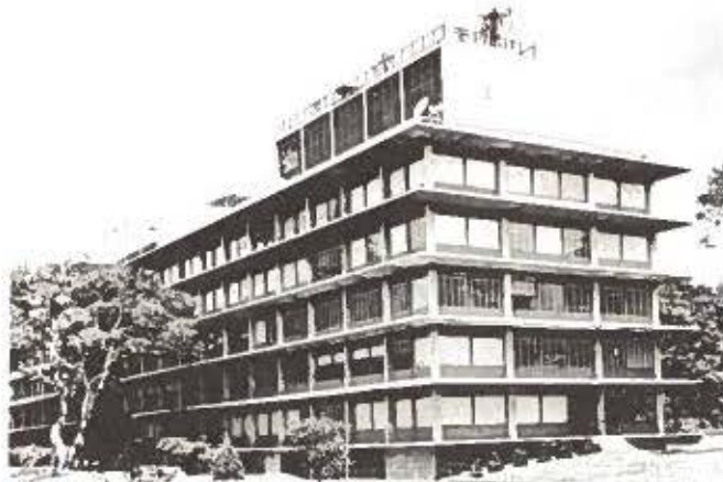
Spanagel Hall, housing the departments of Electronics, Physics, Metallurgy and Chemistry, Electrical Engineering and the Computer Center.
