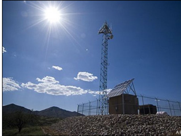
Figure 7. SBNet Sensor Tower
