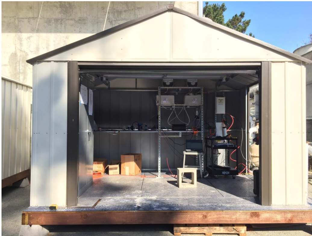
Figure 12. Shed Housing the Hydrogen Production Facility
