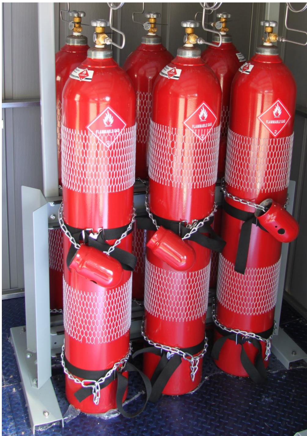
Figure 23. All-Steel, Standard Size, Compressed Gas Cylinders Used for Hydrogen Storage Placed in OSHA, UFC, NFPA, and CGA Compliant Stand with Polypropylene Straps and Steel Chain Straps for Support.
