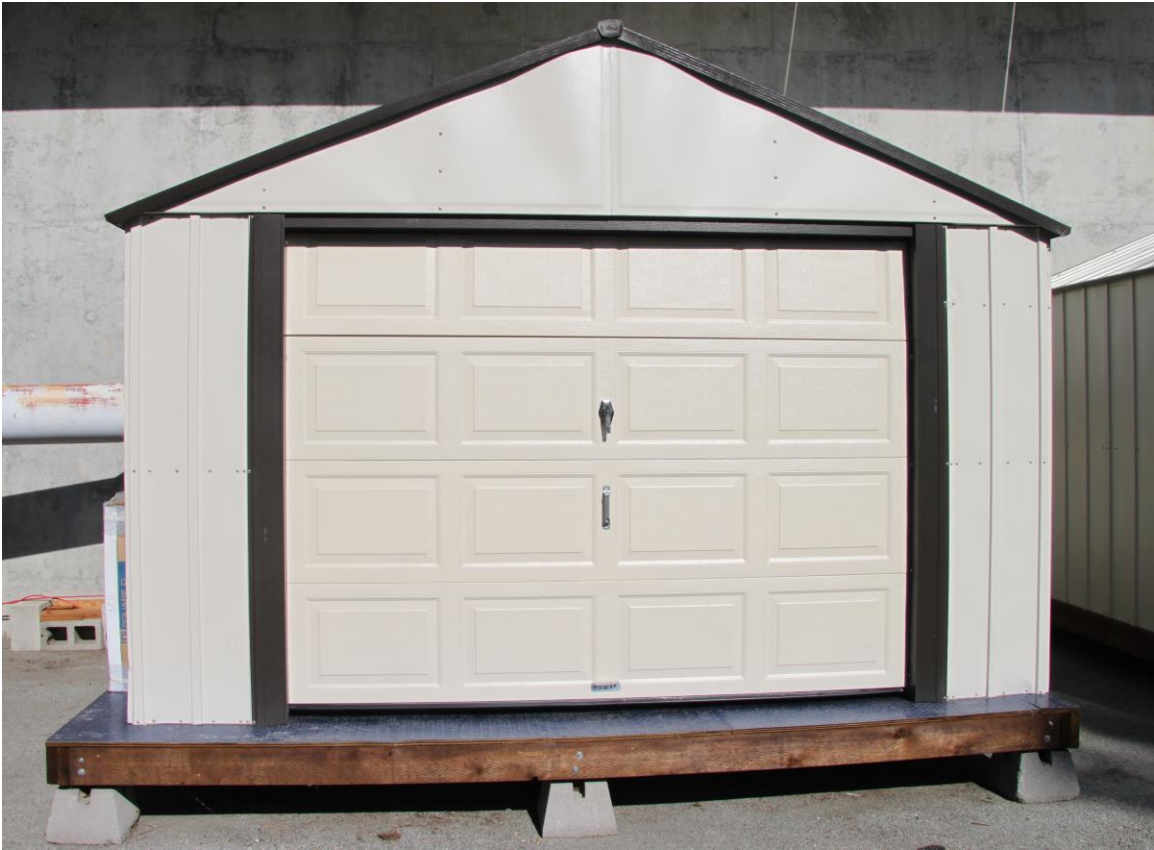
Figure 16. Compression and Storage Station Facility with Weather Protection and Relocatable Platform
