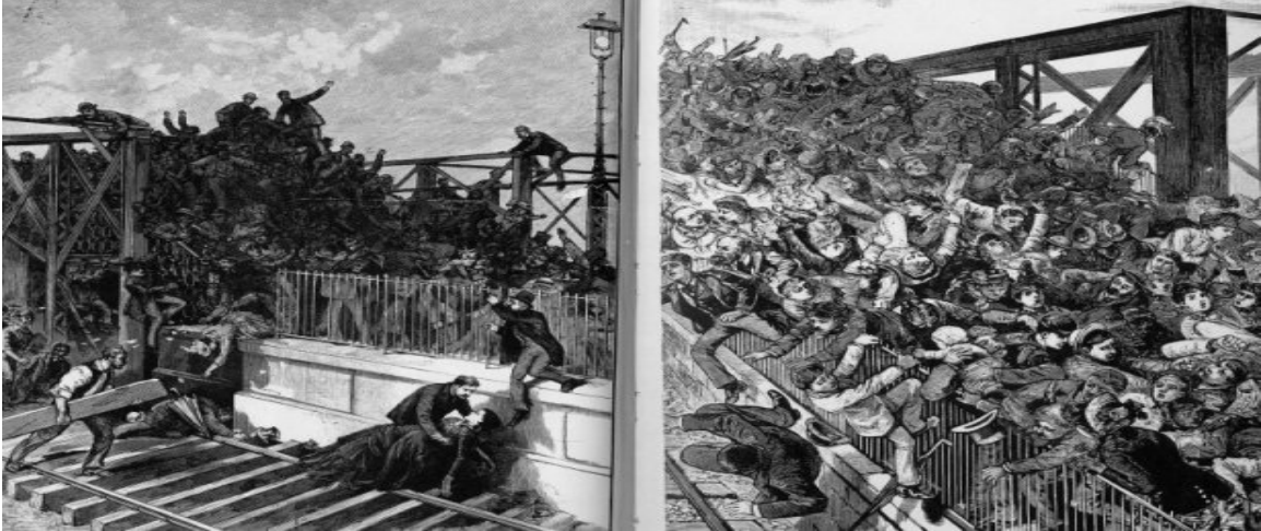
Figure 1. Illustrations of the Brooklyn Bridge Incident 79
