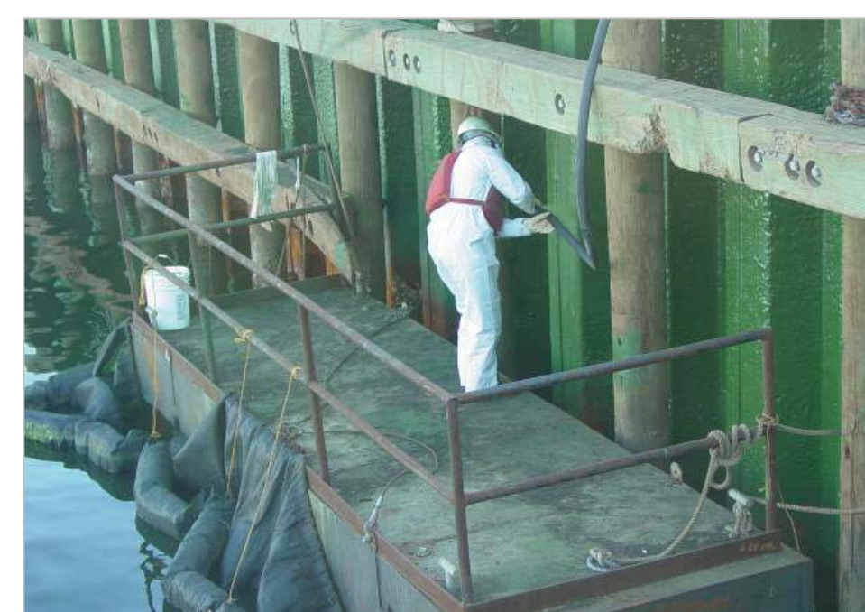
Zero VOC, Coal-tar Free Coating Application at NAS Pensacola, FL
