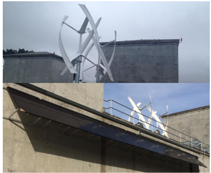
Figure 6. Vertical axis wind turbines and solar panels.
