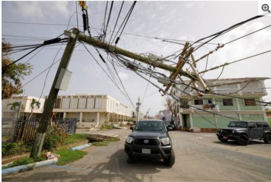
Figure 1.8. Hurricane Maria Damage on STX. Source: Reuters (2017).
