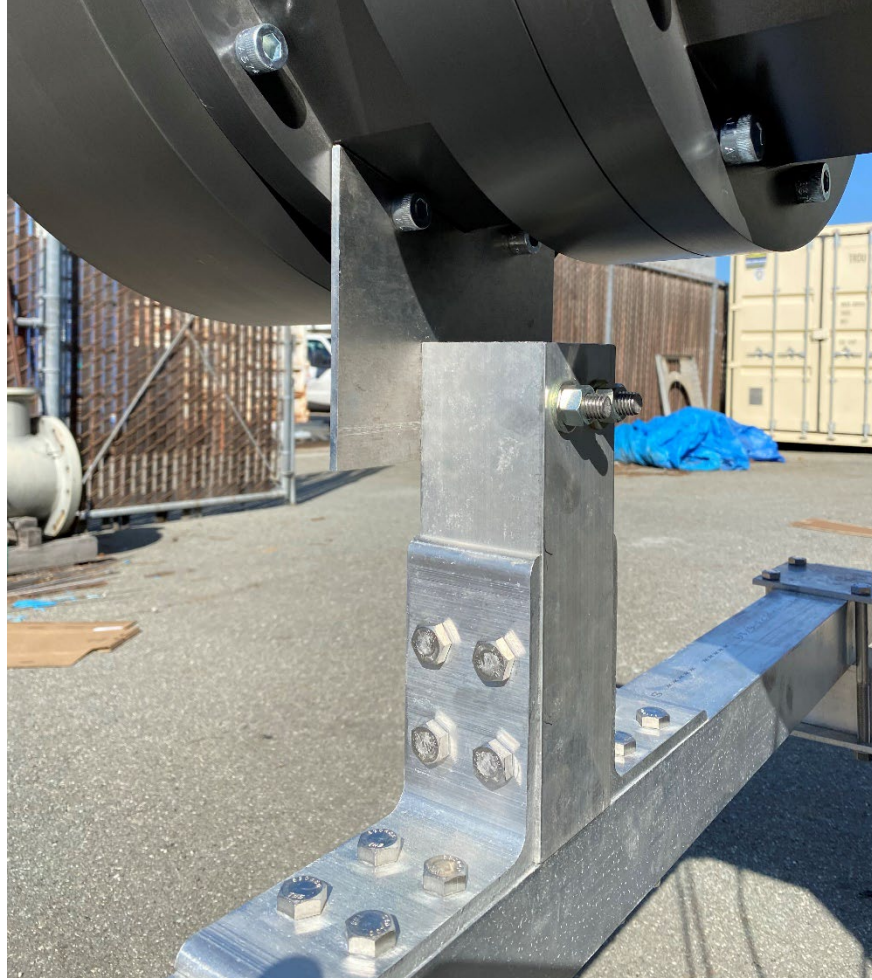
Figure 40. Bell mouth support after installation
