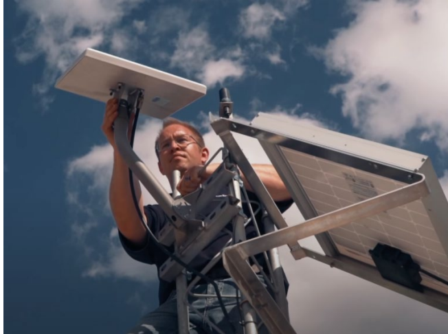
Figure 5. Hughes-branded Inmarsat Broadband Global Area Network (BGAN) M2M Satellite Terminal. Sources: Hughes 9502 BGAN Terminal Brochure (2013) and Asia Satellite (n.d.). Note: The image only shows the outdoor unit (ODU), which is 38.5 cm x 38.5 cm x 3.3 cm. The indoor unit (IDU) containing the modem is an additional 15 cm x 20 cm x 45 cm.
