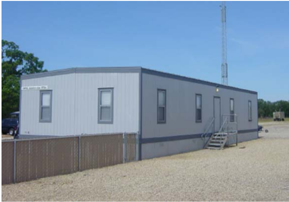
Figure 23. DNOC's Supporting Infrastructure
