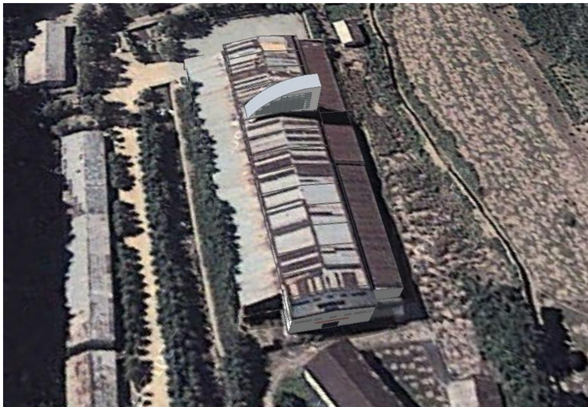
Figure 10 Model of North Korea's Facility to Assemble Transporter-Erector-Launchers
