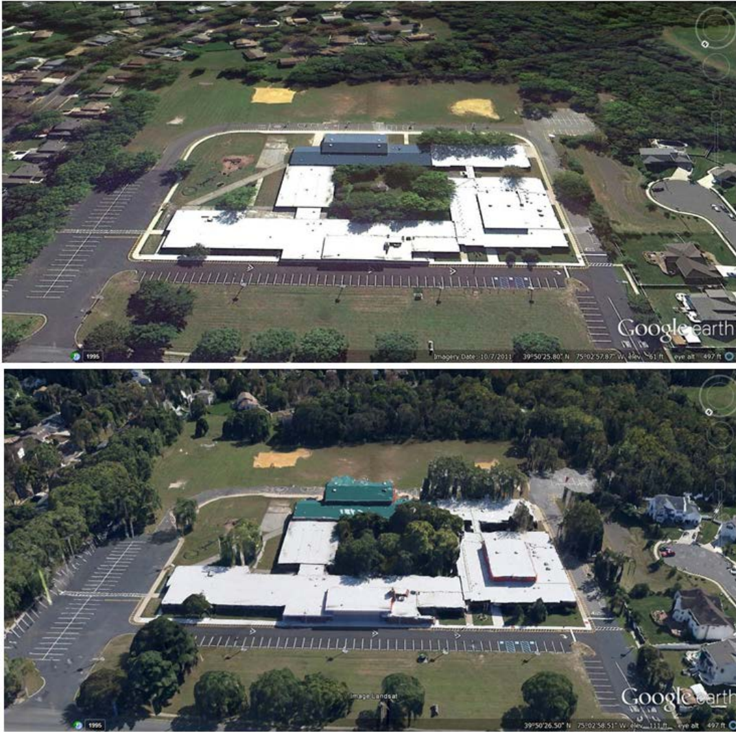
Figure 11. Oblique Satellite Image of School (Top) with 3D Enhancement (Bottom) 84
