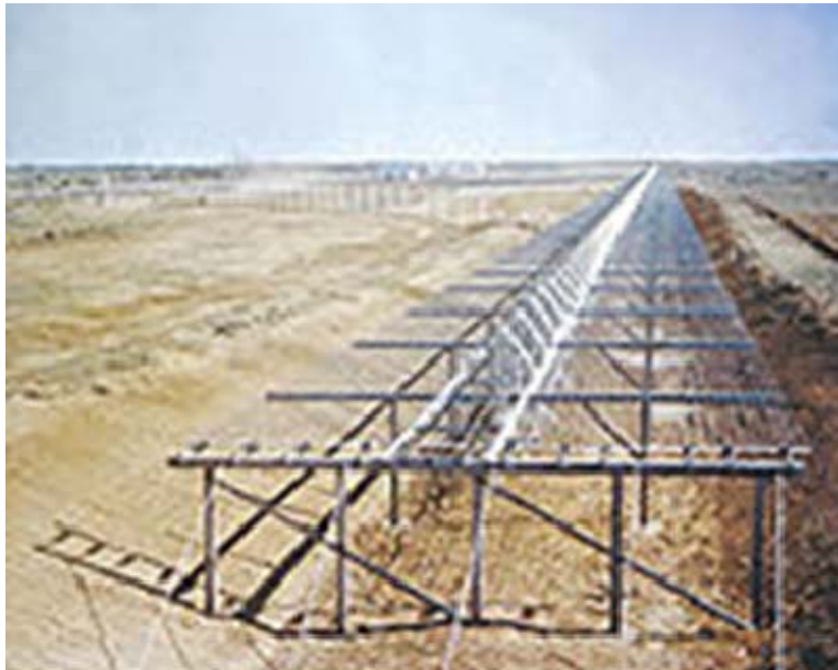
Figure 3. Space Fence (From NAVSPASUR, 2001)
