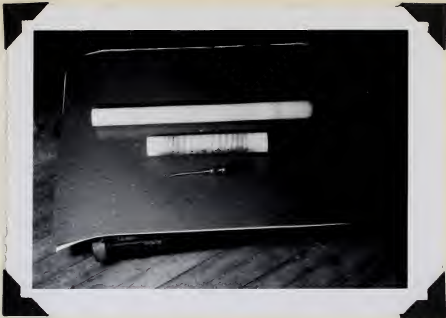
Vitreosil Combustion Tube and Cemented Alumina Combustion Tube
